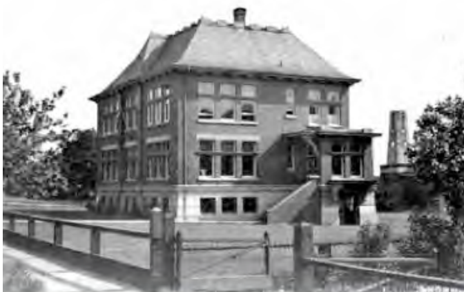
1625 Bank St. Bank Street School. Built by Victoria School Board in 1910-11 to designs by David Cowper Frame. Extant, now used by private school. BCA H-06806/Willis photo c.1930s
